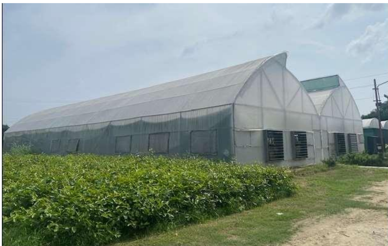
The proposed CPC site is in a nursery complex covering an estimated size of 50 ha.
